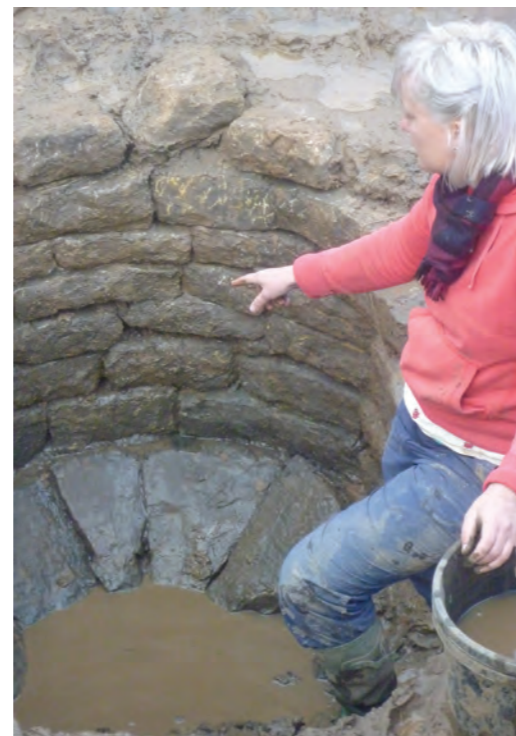
Fig 2.9 Well-laid masonry lining of Well 7, with triangular base slabs partially exposed. © OSA
