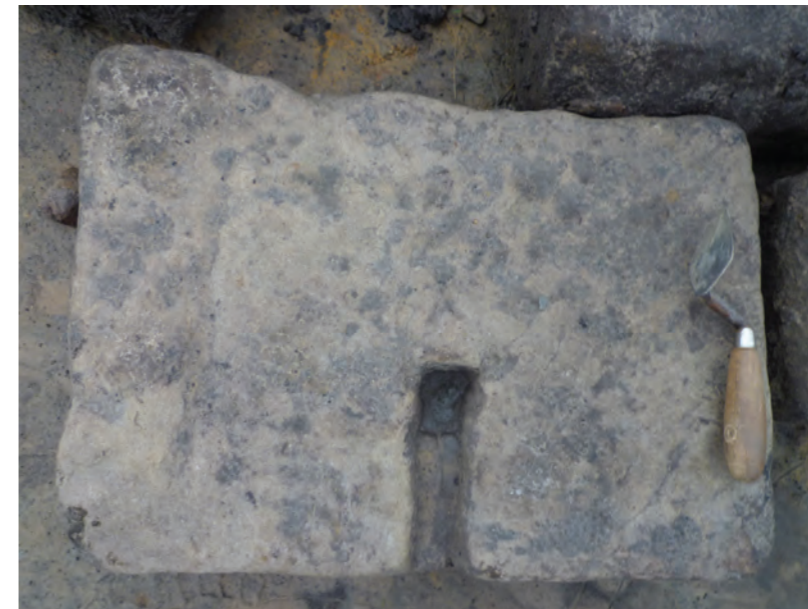
Fig 6.4 One of the stone blocks with features indicative of the opus quadratum construction technique. © OSA
